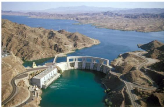
Figure 2.1: Parker Dam at Colorado River
