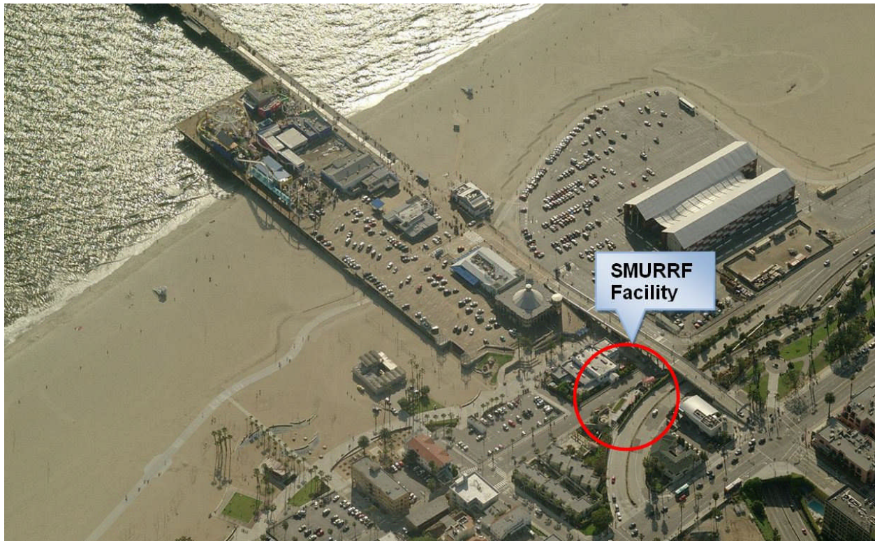
Figure 2.11: Aerial View of SMURRF
