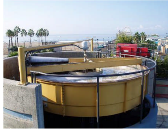
Figure 2.10: Water Treatment at SMURRF Facility
