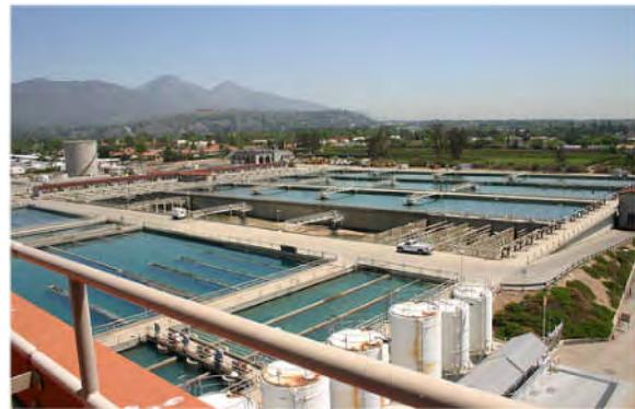
Figure 3.1: Weymoth Treatment Plant
