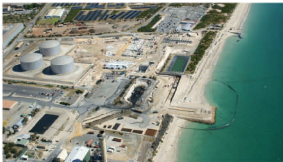
Figure 2.15: Seawater Desalination Plant
