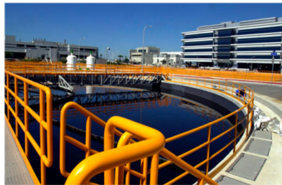
Figure 2.12: Wastewater Treatment at Hyperion
